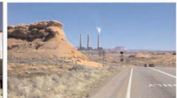
SRP Navajo Generating Plant
