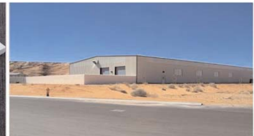
Navajo FlexCrete Plant
