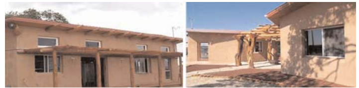
Homes built with the FlexCrete blocks.
