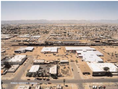
The new Human Services Campus in downtown Phoenix received funding through ADOH programs.
