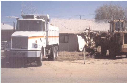
City's Voluntary Demolition Program
