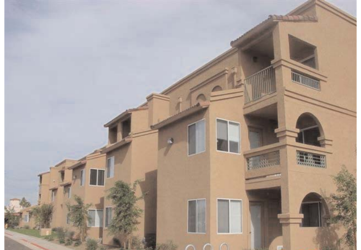
A 72-unit complex developed through ADOH's Low-Income Housing Tax Credit Program during FY2003 opened its doors in November 2003. Homestead Hope, LLC, developed the property, located on West Bola Drive in Surprise. The property will serve households ranging from 20% to 60% of the area median income, with the majority of units reserved for populations earning 50% or less of area median income.
