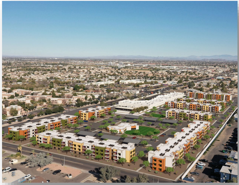
Centerline I and II: Glendale, AZ
