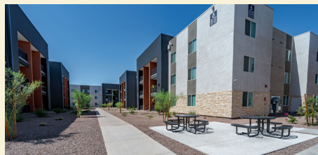
Salt River Flats – 192 Units (Phoenix)
