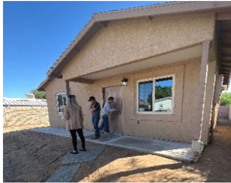
Yuma County - Colonia Home Rehab Project (After)
