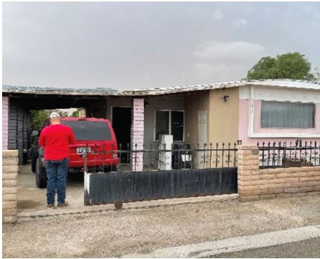
Yuma County - Colonia Home Rehab Project (Before)
