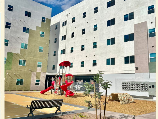
Mesquite Terrace – 297 Units Phoenix
