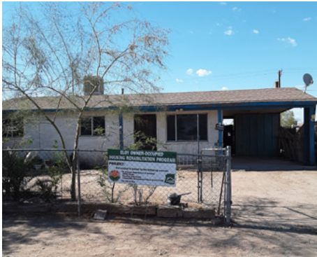
City of Eloy Home Rehab Project (Before)
