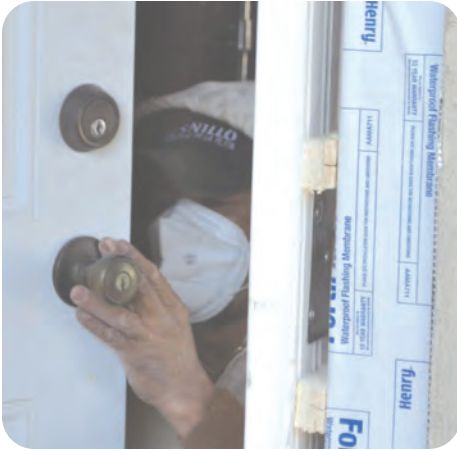
7. Ensure door is fully operational and lock set is aligned
