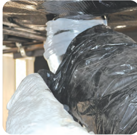
2. Pull insulation over hard connections as needed
