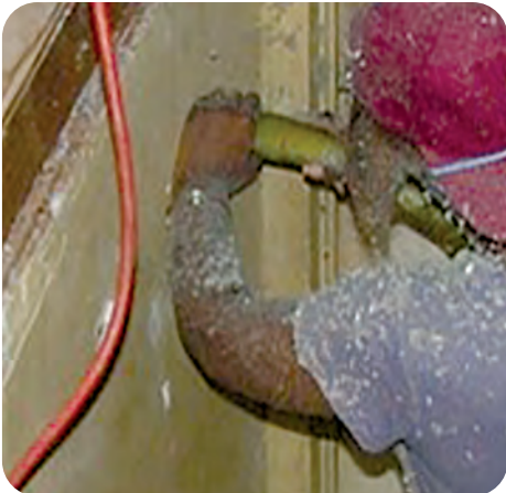
7. Dense pack stairway walls
