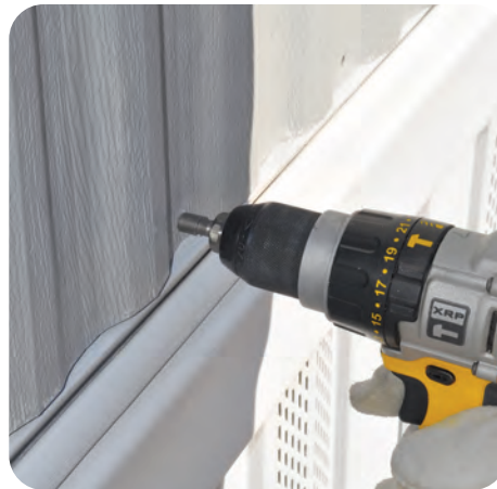
9. Reattach mechanical fasteners
