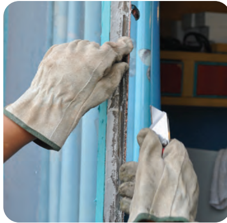
2. Clean all debris, caulk, etc., from sash
