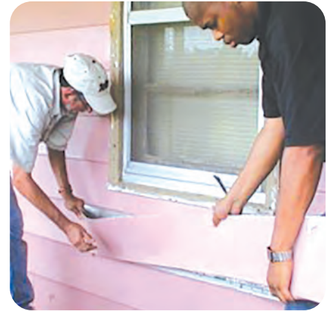
9. Replace and/or repair siding
