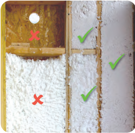
7. If possible, ensure all cavities are filled before completing job
