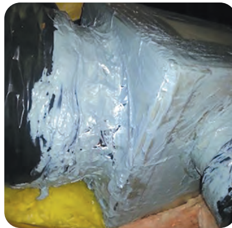
4. Seal new joints
