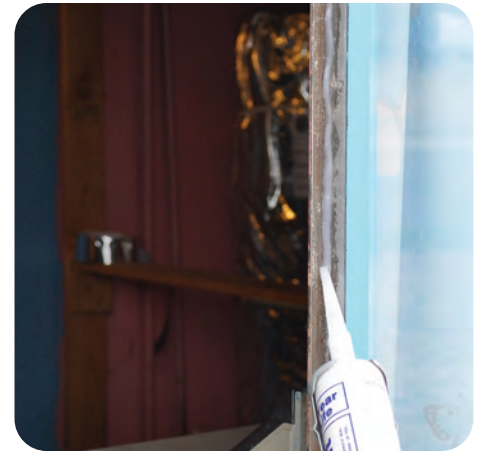
4. Run interior bead of caulk
