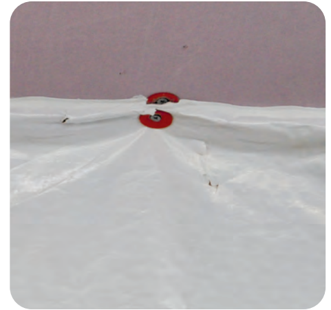
3. Seal seams of belly wrap
