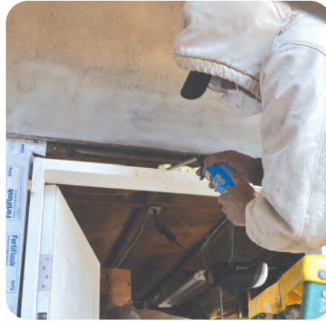
8. Insulate gaps between door jamb and frame
