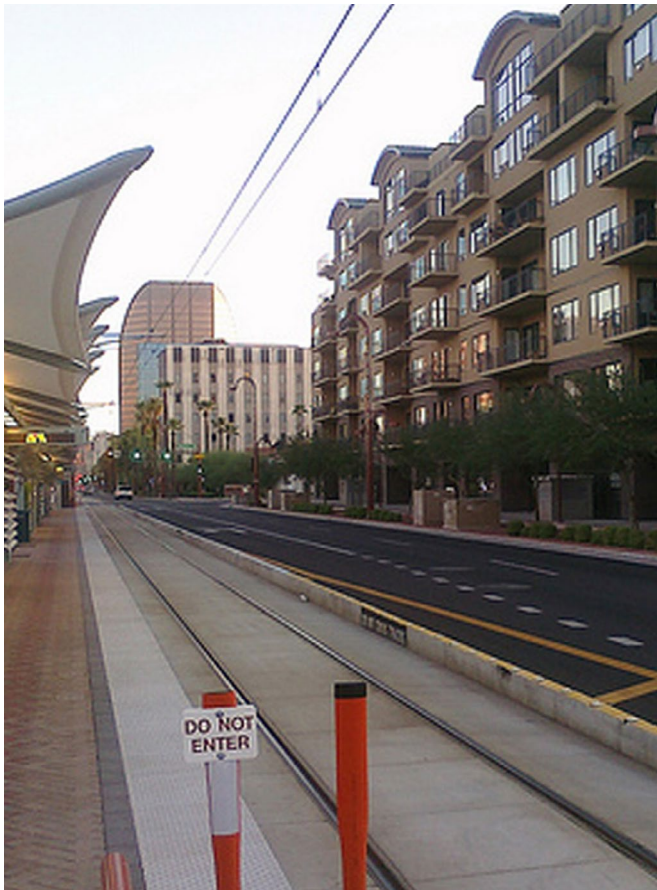
Tapestry Luxury Condominiums, Central and Encanto Blvd. Phoenix, Arizona Source: http://raillife.com
