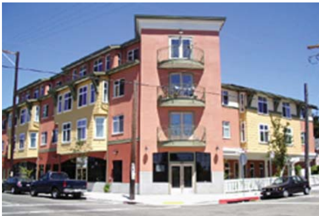
This affordable housing complex in Berkeley, California serves seniors with household incomes less than 30%, 50%, or 60% of the area median income. Source: bbiconstruction.com
