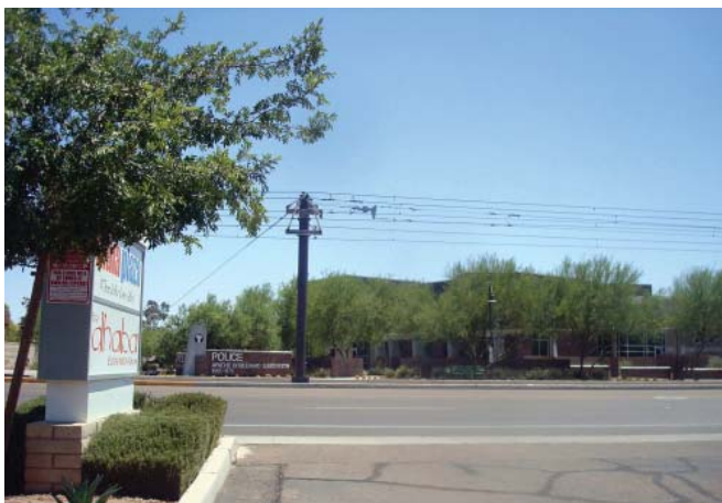
Apache Boulevard Police Substation
