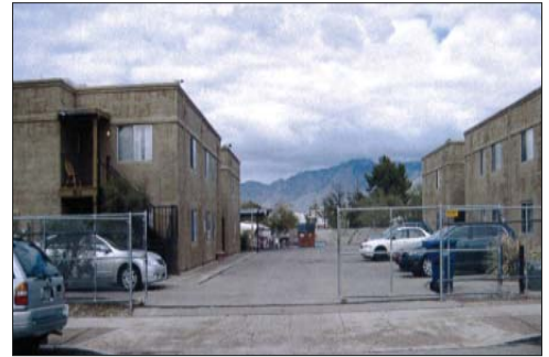
Vida Nueva Apartments before rehabilitation,
