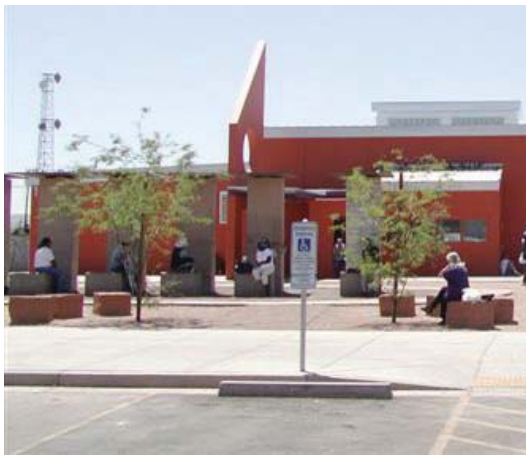
▲ Lodestar Day Resource Center serves as a one-stop shop for homeless services on the Human Services Campus.
