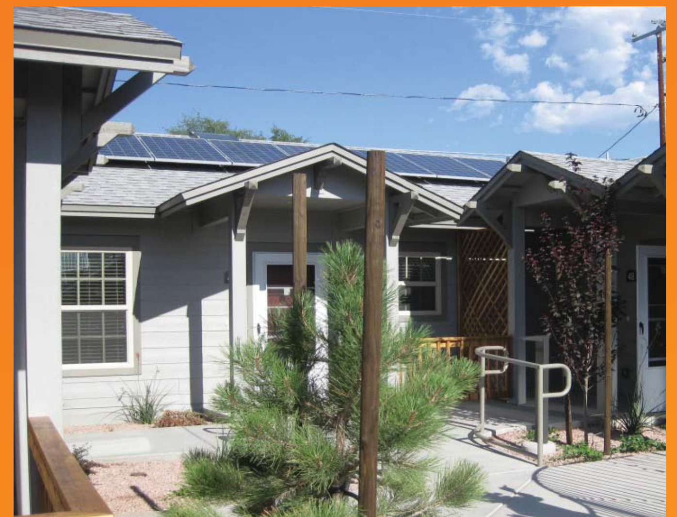
Pineview's residents are proud of the "green technology" the solar panels on their roofs represent.
