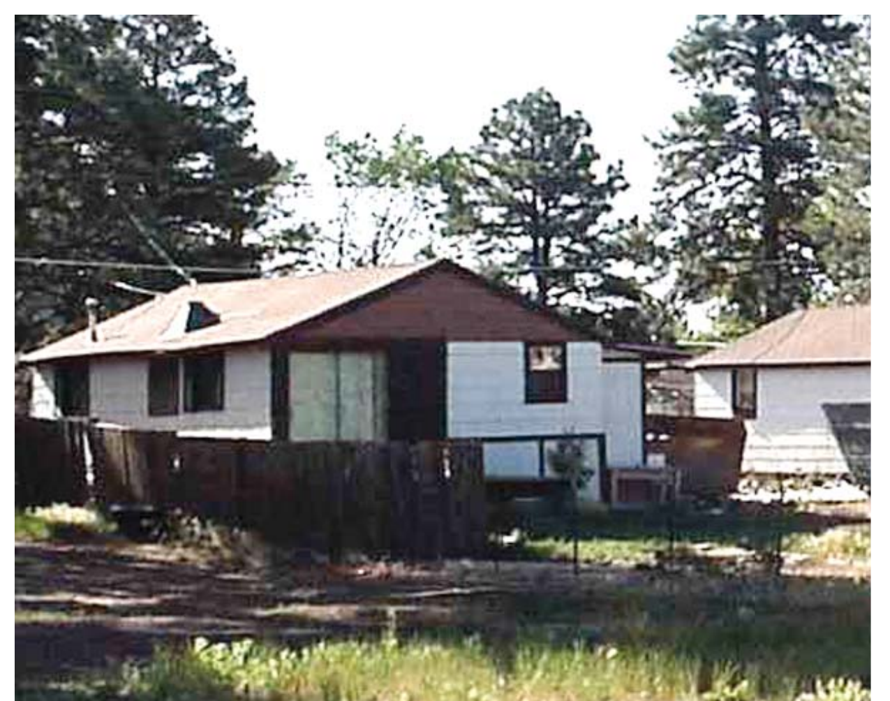
This property (middle photo) has been razed and is now under construction (bottom photo). The project, while already planned before the City of Flagstaff Community Housing Policy Task Force was implemented, incorporates many of the recommendations outlined by the Task Force.
